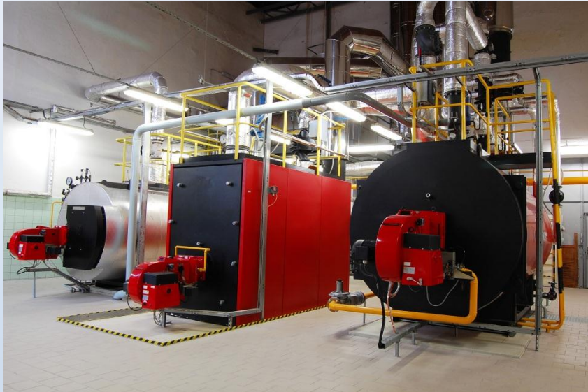
Modern steam boilers benefit from water quality monitoring
