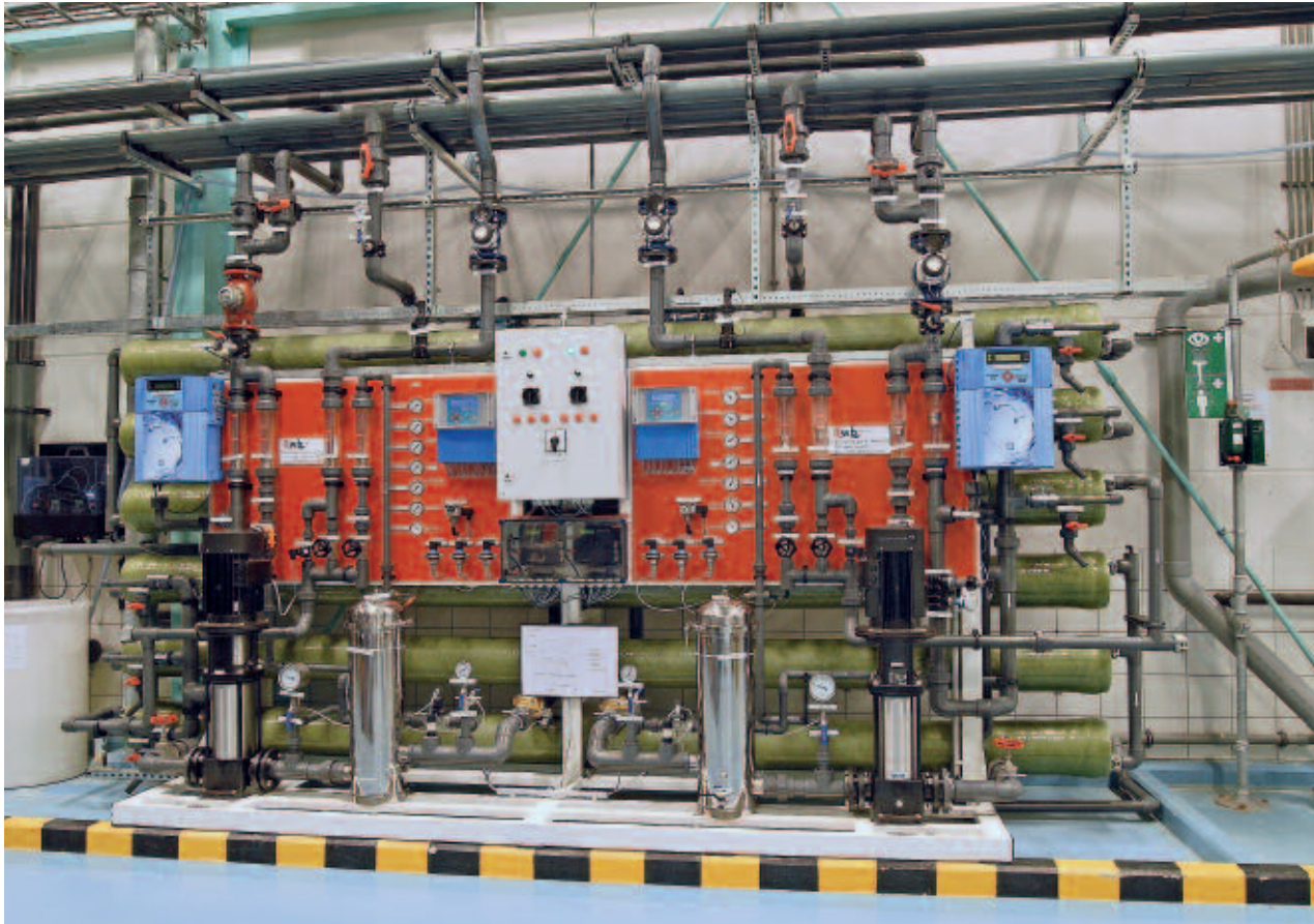
Nano filtration plant with integrated Testomat® instruments and Softmaster® controllers in a Dutch food processing company
